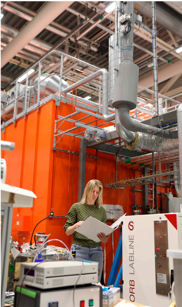
At the buffer system that helps securing toxic gas waste in the facility.
