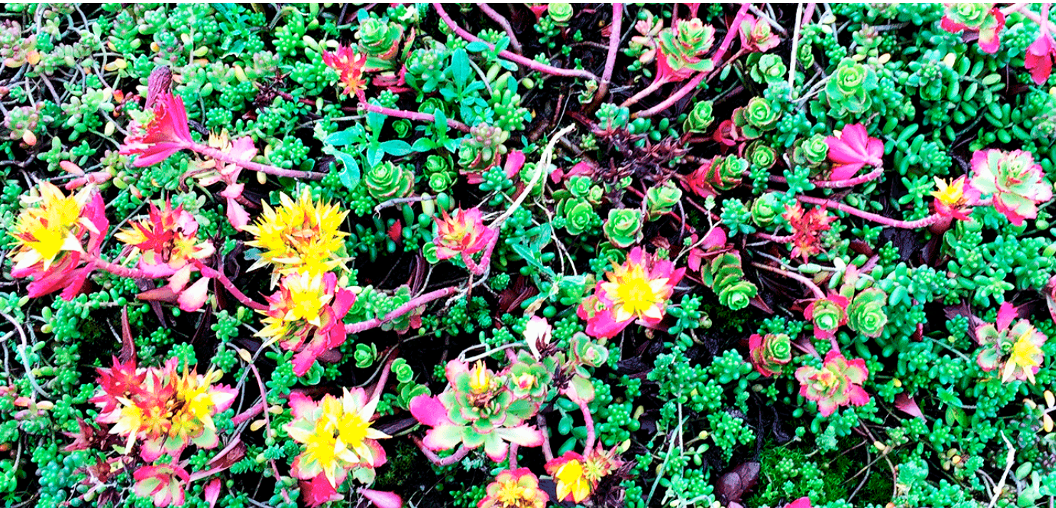
Close-up of the green roofs at MAX IV which improve insulation, help stabilising the temperature in the experiment halls while storing and delaying rainwater drainage to reduce the impact on sewage systems, and improve wildlife environment.
