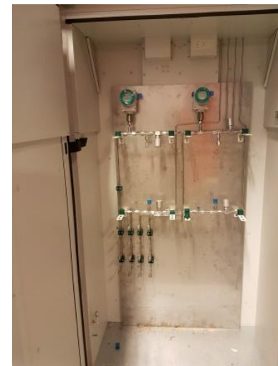
Gas mixing panel and gas cabinet
